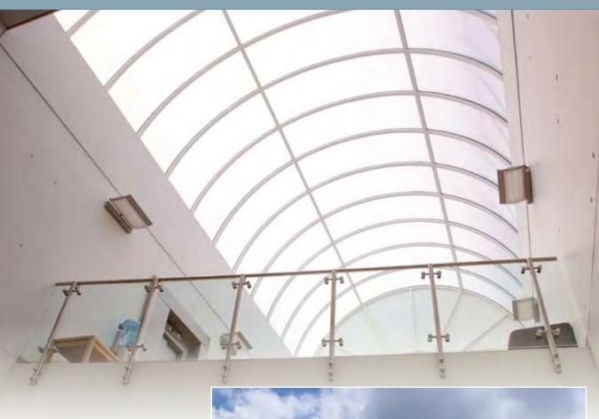
The classic vault is a simple semi-circle that tops the supporting structure. Aalternatively, it can be extended on vertical legs incorporating such features as windows, vents or louvres. Ends can be terminated with vertical glazed screens or simply abut an adjoining structure.
