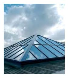
Illustrated here are details from a selfsupporting pyramid installation, designed and constructed with 30° geometry and set into a flat roof.
